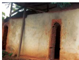
Earth brick kiln-Daboase (INBAR)
